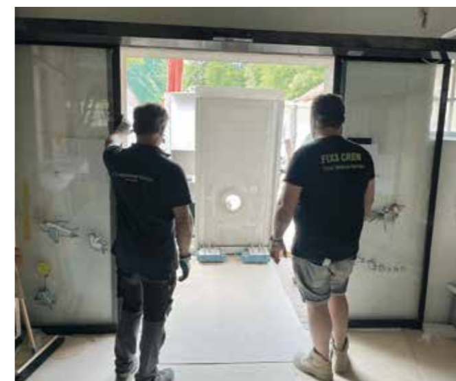
Exactly two centimetres of space in each direction was enough to push the sledge with the aquarium, which now weighs more than three tonnes, through the door and into the house.
