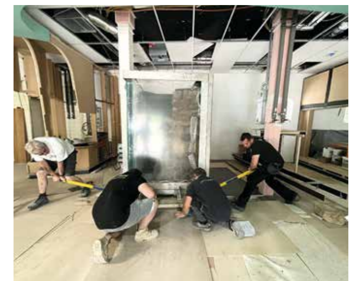
The aquarium needs strong men. In the end, the part was centimetre-perfect in the right place. Only then were the acrylic discs glued in and sealed.
