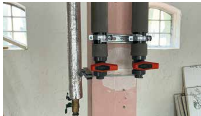
End of March: the pressurised water pipes for osmosis water and mixed water pipes to the individual modules as well as the ventilation ducts are laid, the ceiling can be partially sealed.
