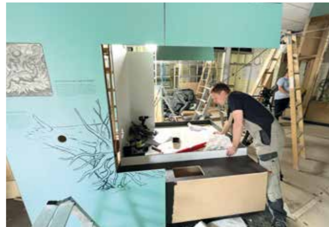
Each individual module had previously been completely assembled and disassembled in the joinery to check the accuracy of fit. Each of the visible panelling panels is glazed several times and then printed by the print shop in a multi-stage process.
