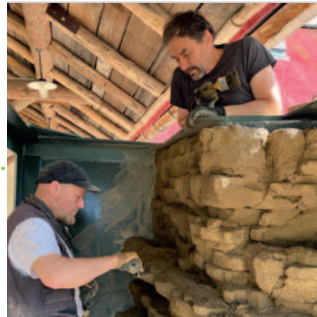
Artificial rock builders Andreas Gehlen and Oliver Blomeier installing riverbank embankments on Lake Titicaca.
