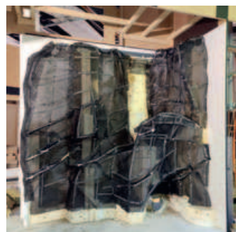
... which is covered with a mesh to hold the artificial rock in place. | Oliver Blomeier
