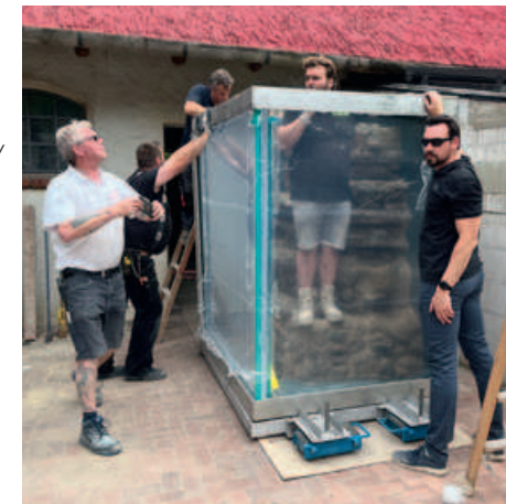
After inserting the pane, the upper steel frame is placed on top and screwed into place. Now everything is ready and we can get started.
