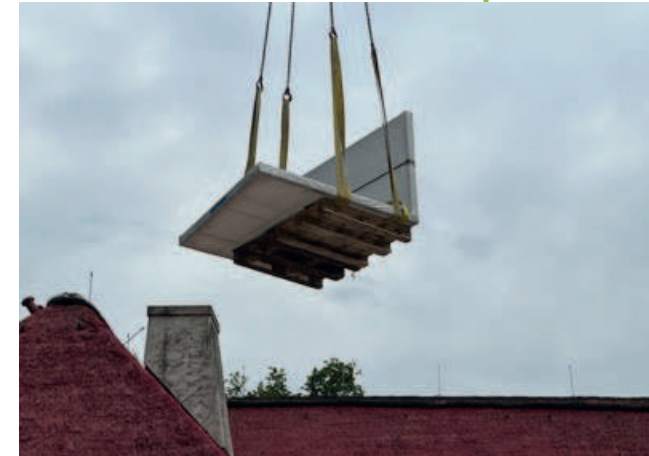
Before that, the acrylic glass pane arrives from South Korea via Rotterdam and is installed.
