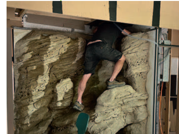
Water test: The rock is reworked until the water from the surge tank at the top runs down the rock in the right places.
