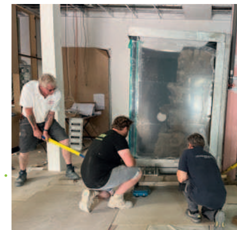
The tank slides into the room without a scratch on the door arch. The final challenge is to position it exactly. Here, every centimetre counts to ensure a precise connection to the exhibition octopus.
