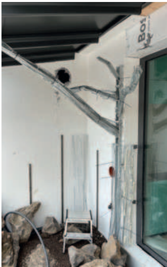
An artificial rock tree is integrated as a design feature to separate the exhibition area. Its 'board roots' flow around the natural boulders between which it 'grows'.
