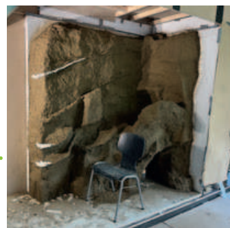
The artificial rock is sprayed on in several layers.
