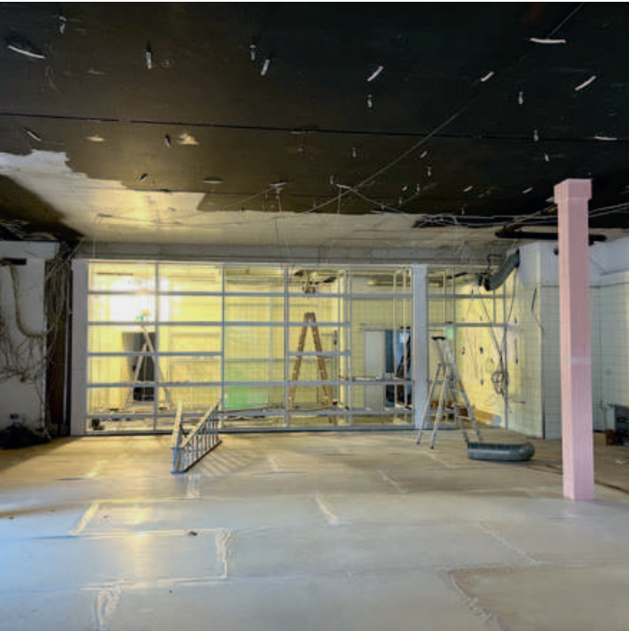
The first thing to be installed is the shelving for the future breeding area.
