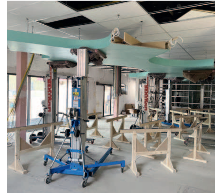
The entire module will be assembled and lifted by hand to the ceiling as a whole.
