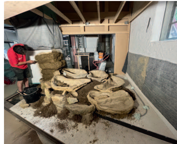
In June 2023, the first artificial rock structures, the tubs for the toad enclosure, will be manufactured individually, positioned on the site and connected to each other.
