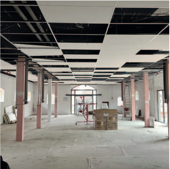
By March 2023, most of the pipes will have been laid under the ceiling.
