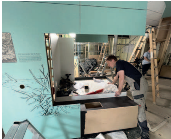
Interlocking trades: Part of the cladding on the Fire Salamander module is in place, now half of the basin has to be fitted and the artificial rock tree designed before the basin and cladding can be completed.
