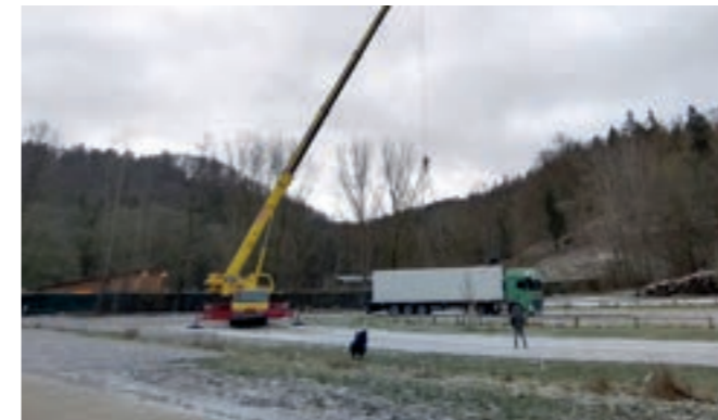
Delivery of the container to Hundshaupten, where it was hoisted into position over trees, a stream and a wall in freezing temperatures.
